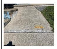
23. Remove asphalt and replace asphalt with concrete of the same form 25sf.
