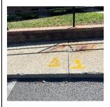
2.Grind curb and panels to eliminate trip hazard 10ft
