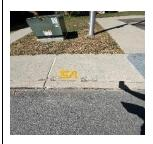
5B. Patch curb Cut, remove and replace 2 ft section of curb.
