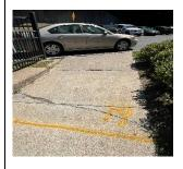
20. Grind trip hazard, caulk seam 5ft
