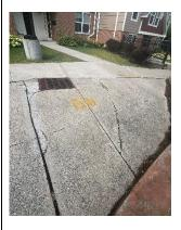
14. Patch wall at stairs with concrete (no additional blocks), patch stairs, grind trip hazard at top - grind 5ft
