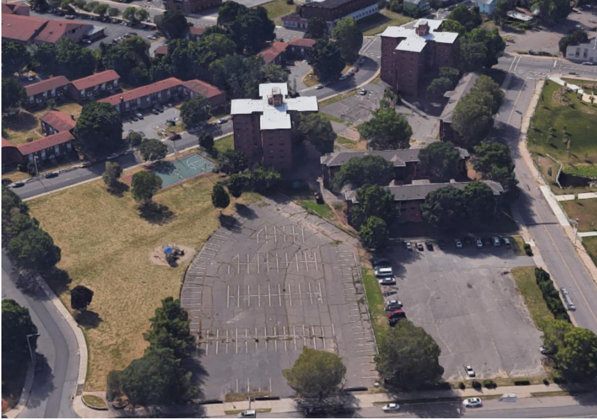
Before: Super block with Meriden Mills low and high-rise public housing apartments
